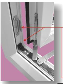
Fit Stay Guard Elite approx 75mm centres from the internal corner as show here. Secure using 4.8 X 25 carbon steel zinc coated screws
